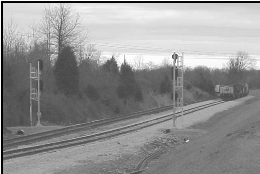
New south switch at the extended siding at Kelly on CSX's Henderson Sub. Note also the new signals. Kelly, KY February 7, 1999.
